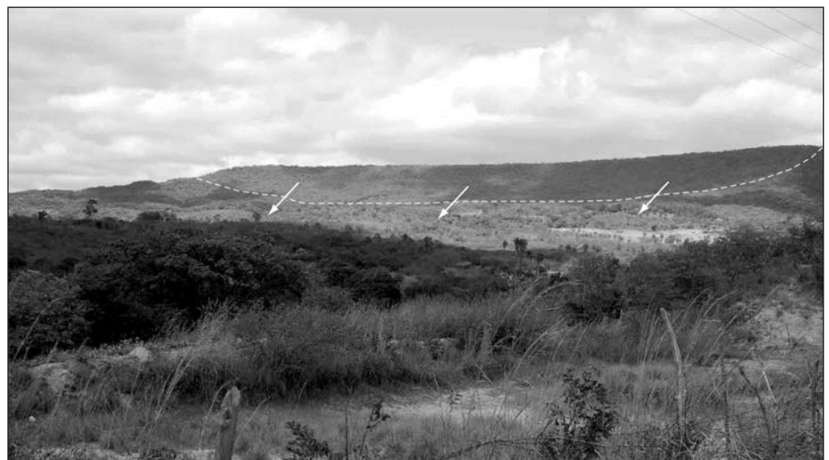
Fig. 11 – The Carretão landslide scar, south of Crato. Photo: J.-P. Peulvast.
